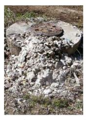
Figure 42: Grease interceptor overflow.
