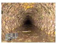
Figure 2: FOG accumulated on the wall of sewer pipe.
