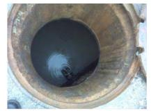
Figure 28: Cleaned interceptor.
