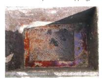
Figure 33: Grease interceptor not working.
