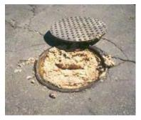
Figure 22: Interceptor filled with grease to the top.
