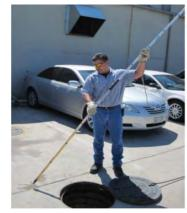
Figure 25: Inspecting the interceptor.
