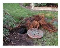
Figure 35: Roots removed from the grease interceptor (root intrusion can completely clog the interceptor).
