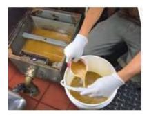
Figure 19: Removing grease from the grease trap.
