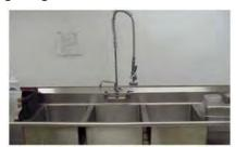
Figure 7: Three-sink dishwashing system.
