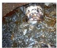
Figure 38: Missing inlet tee allows FOG buildup in front of discharge pipe.
