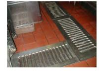
Figure 9: Floor drain screen.
