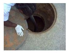
Figure 26: Vacuuming out the contents of the interceptor.
