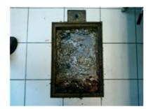
Figure 43: Grease trap overflow is a hazard to kitchen employees.
