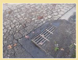
Standing water due to clogged drains can damage pavement.
