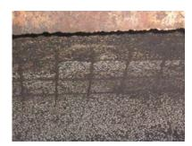
Figure 37: Exposed re-bar in a corroded concrete interceptor.
