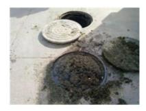
Figure 41: Grease interceptor completely full. Heavy lids can be lifted up under pressure and grease start overflowing.
