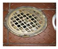
Figure 30: Debris in the floor drain (floor was not swept before mopping).
