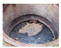
Figure 39: Missing outlet tee allows floating FOG to escape into the sewer system.
