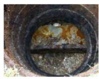
Figure 34: Too short outlet tee allows short-circuiting.
