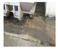
Figure 32: Waste leaks in the garbage and grease recycle storage area.
