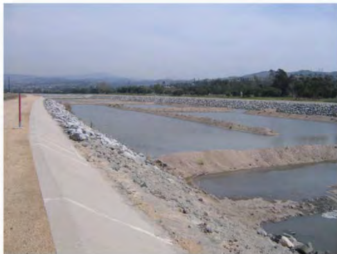
FIGURE 4-5 SAND LEVEES IN THE SANTA ANA RIVER
