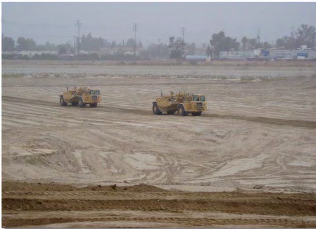
FIGURE 4-6 CLEANING OF RECHARGE BASINS
