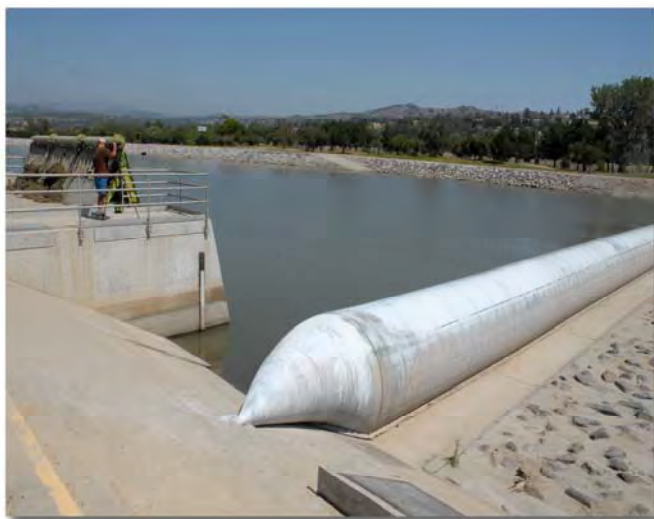
FIGURE 4-4 INFLATABLE DAM ON THE SANTA ANA RIVER
